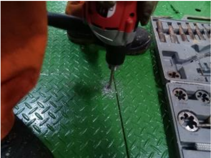
Drill through the plate and the frame bar.
