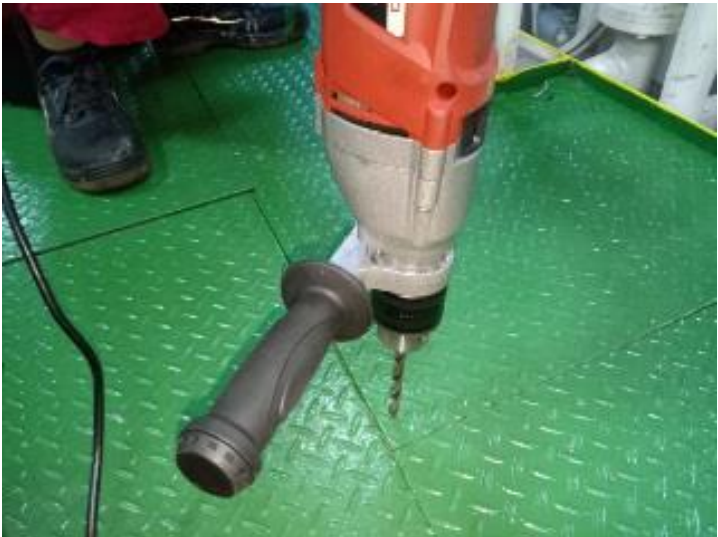
Drill through the plate and the frame bar.
