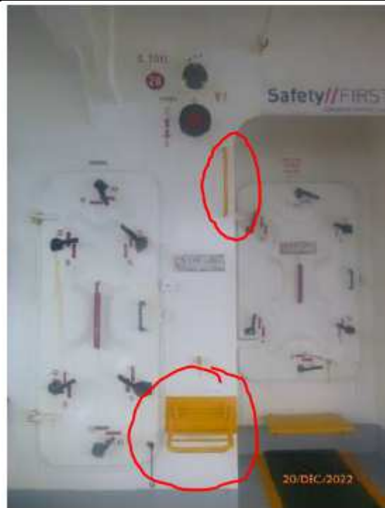
Step and hand hold installed on bulkhead
